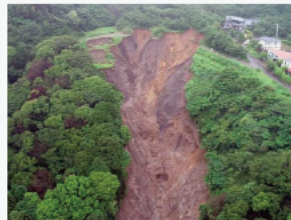
2021 Atami embankment collapse (from Shizuoka Prefecture)
