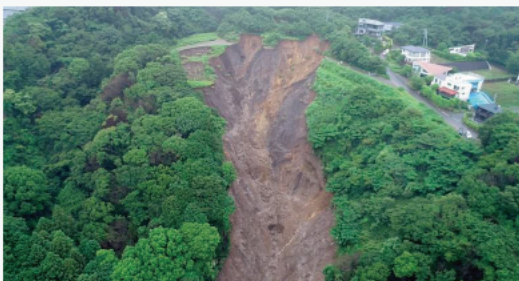
Embankment collapse at the head of Aizome River Shizuoka Prefecture UAV photograph (July 3, 2021)
