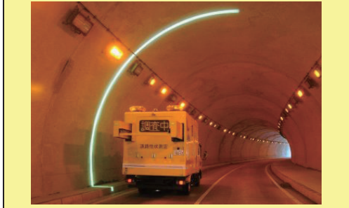
I . The captured image of the tunnel
