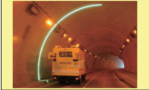
I . The captured image of the tunnel
